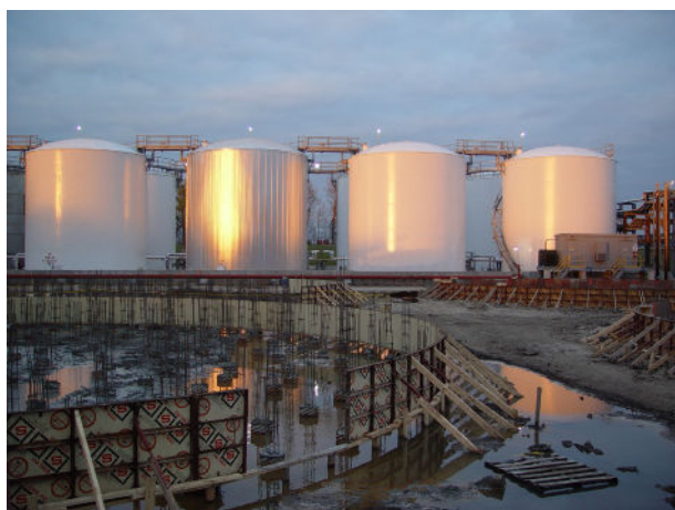
Figure 4. AT&V's construction of pressurised storage for hydrocarbon terminals.
