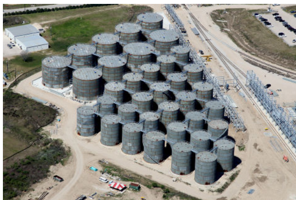
Figure 5. Typical atmospheric storage facility featuring 36 tanks built by AT&V.
