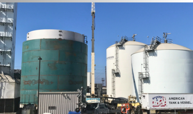
Civil, tanks, and painting 5 months, no overtime
