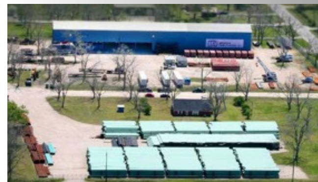
Houston export/fabrication plant
